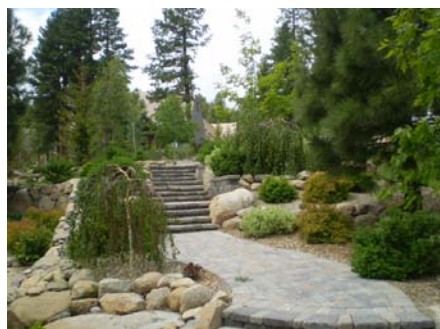
PHOTO #32 NO HAND RAILS AT ENTRY STAIRS, WEST
