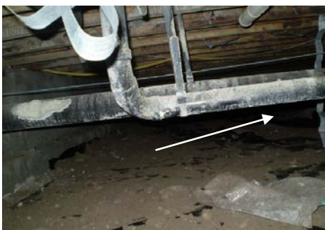
PHOTO #15 UP HILL SLOPE OF WASTE LINE BELOW WEST BATH
