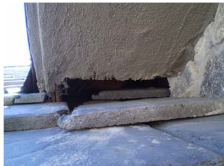
PHOTO #28 OPENINGS UNDER EAVES ARE OPEN TO ATTIC. ACCESS FOR BIRDS AND ANIMALS
